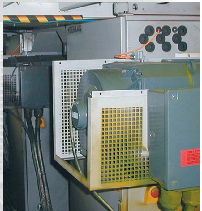
Monitoring of the overall vibration of rotating components.
